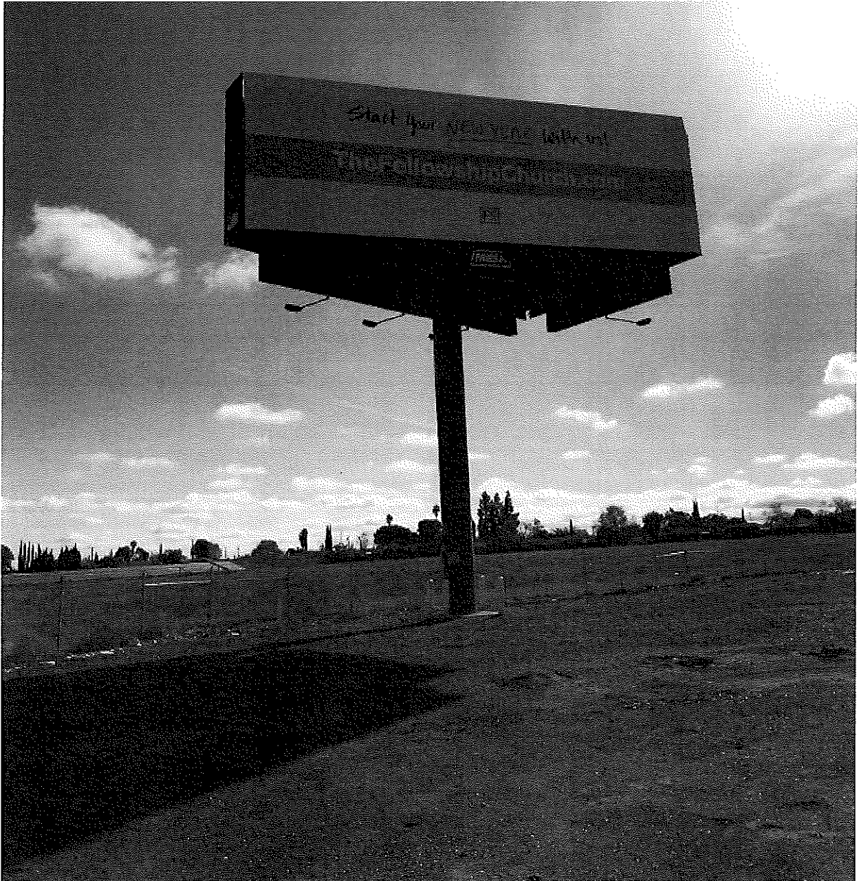
Facing East towards the West face that will be upgraded, January 23, 2018
