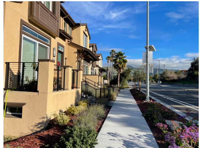
Landscaping buffer between the sidewalk edge and the building edge along a primary street frontage.
