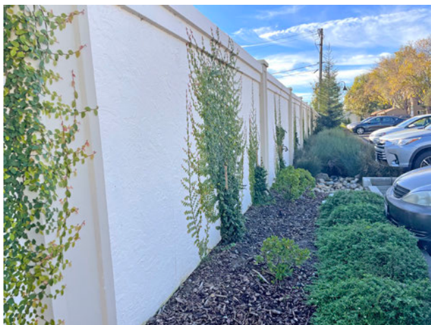
Perimeter wall with decorative columns and landscaping to break up and soften its appearance.
