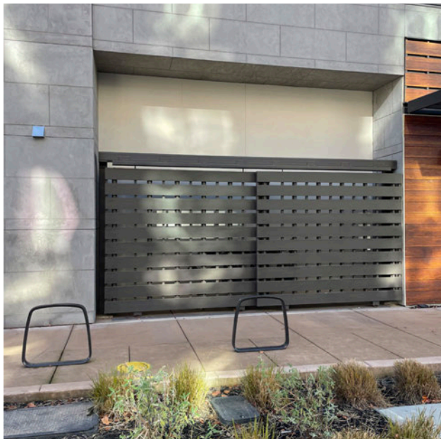
Trash area screened from public view with fencing and gate of matching material and color.
