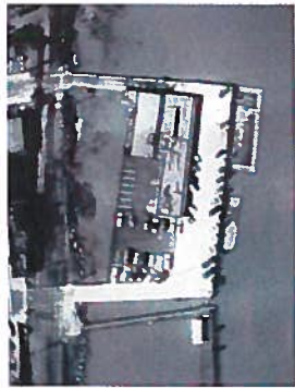
Photo 2.6 – Downtown Riverview Pier - Previous Riverview Pier Deck (Date Unknown but assumed 1966 or later)
