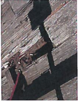
Photo 3.24 – Downtown Riverview Pier - Pier Timber Deck
