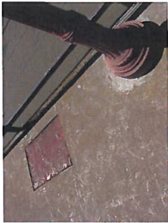
Photo 3.38 - Downtown Fishing Pier - Main Pier Deck Slab
