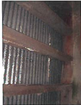
Photo 3.19 – Downtown Riverview Pier - Pier Deck Stringers
