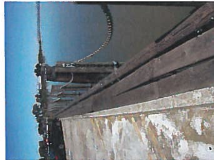
Photo 3.28 – Downtown Riverview Pier - Pier Frontage Decking Missing
