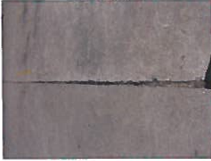
Photo 3.22 – Downtown Riverview Pier - Pier Concrete Deck Joint
