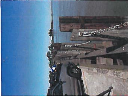
Photo 3.28 – Downtown Riverview Pier - Pier Frontage Decking Missing
