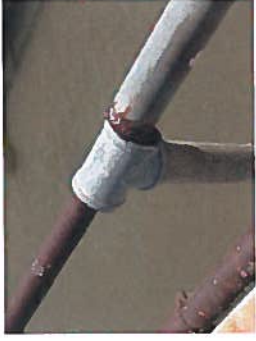
Photo 3.26 – Downtown Riverview Pier - Pier Handrails
