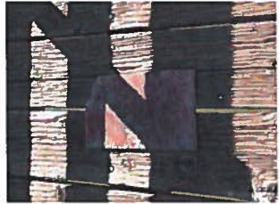
Photo 3.8 - Marina Fishing Pier - Pier Deck Patch
