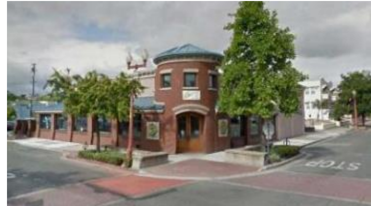
Figure 2.2.4: SW Corner of G Street at 4 th Street
