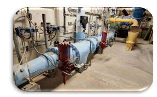
Project Description: This project will replace four aging filter valves in Plant 'A' at the Water Treatment Plant.
