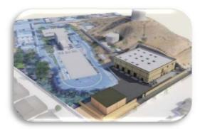
Project Description: This project will construct a 6 MGD brackish water desalination plant that would treat water from the San Joaquin River during times of high chloride content. The work will include the replacement of the City's river intake facility and install a new fish screen. Approximately 4 miles of pipeline will be constructed to convey brine concentrate from the water treatment plant to Delta Diablo.
