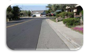
Project Description: This program prepares roadways to receive a full street width surface treatment such as a cape seal or micro-surfacing by constructing asphalt concrete plugs and leveling courses typically within the driving lanes.
