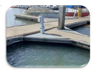
Project Description: This project will replace the docks, floats, and slips at the Marina. Assessments of dock conditions and dive survey to assess the floats will need to be conducted and corner board of slips should be replaced with newer Ultra High Molecular Weight Polyethylene plastic boards.
