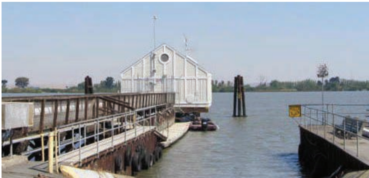
Figure C-1. River Pumping Station is constructed on pier above the San Joaquin River. The PS needs interior renovation and some improvements to the discharge pipeline.
