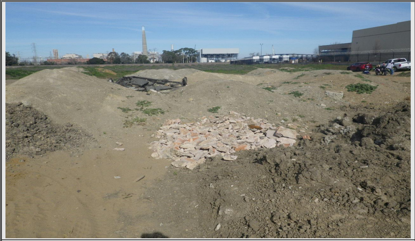
Photograph 36 – View of Concrete & Asphalt, Northern Portion of Parcel 56, 3215 E. 18 th Street
