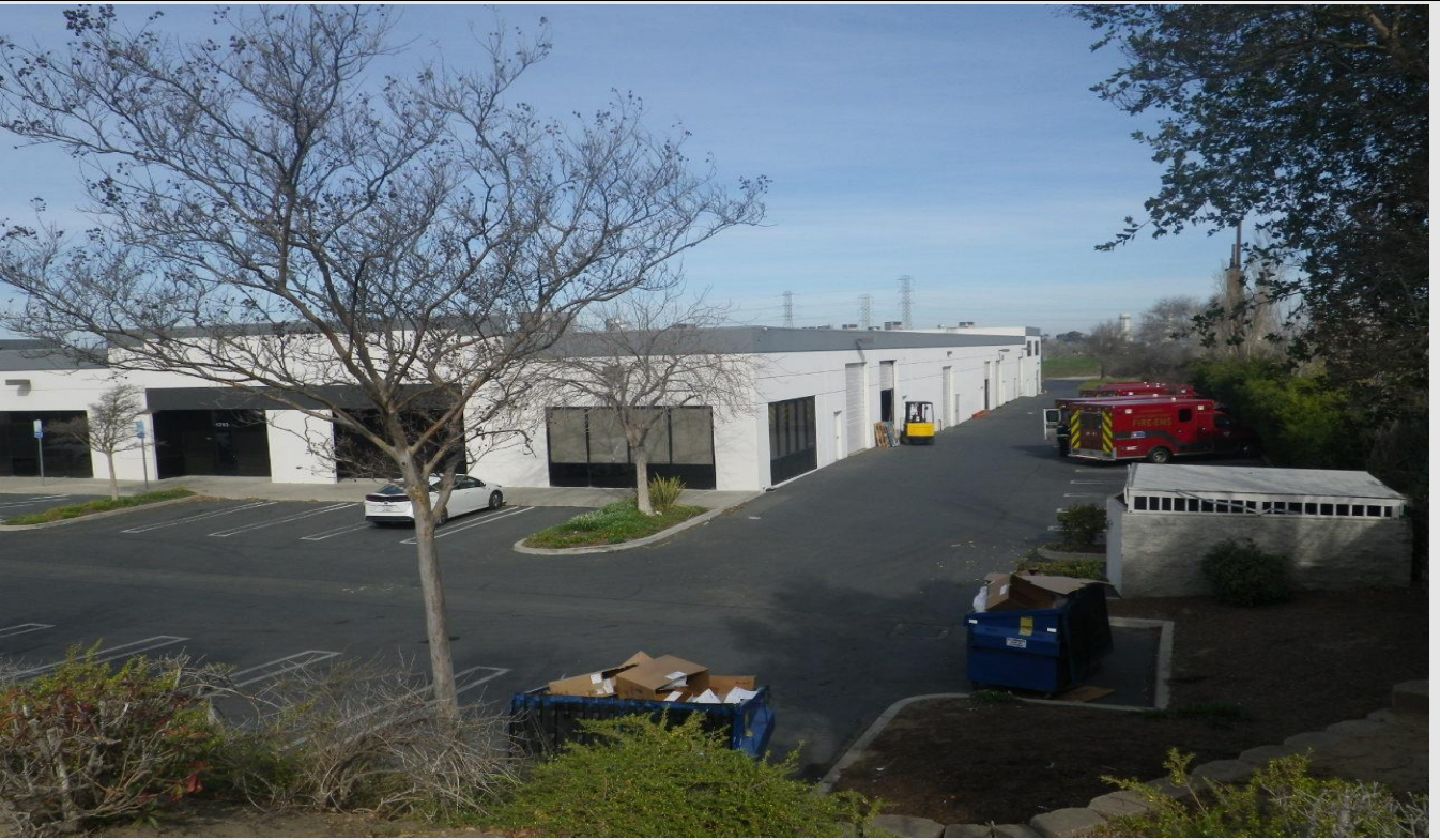
Photograph 22 – View of East Side of Vineyard Business Park, Parcel 102 (1793 Vineyard Street)
