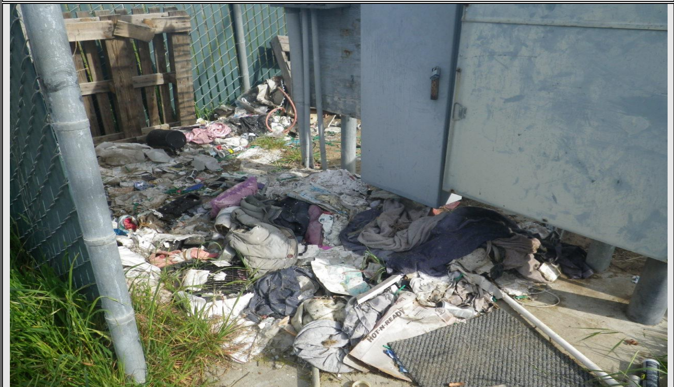
Photograph 30 – View of Trash in Water Tank Compound, 2901 E. 18 th Street, Parcel 86
