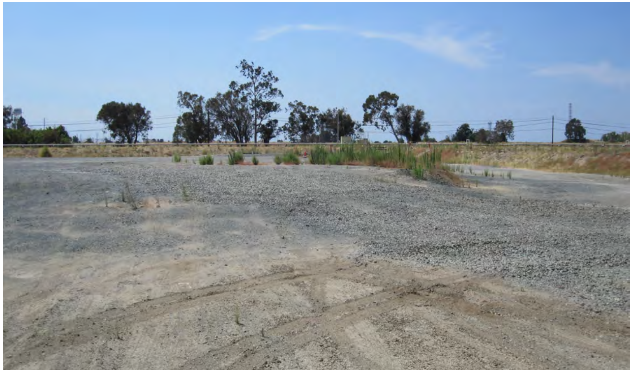
Photo 5B: Looking west over the northern edge of the middle tank pad. The earthen dike in the background will be regraded. The asphalt tank pad is covered by a thin veneer of soil and gravel. Trees dominant in background are the same as those shown in Photo 4C and will be removed.
