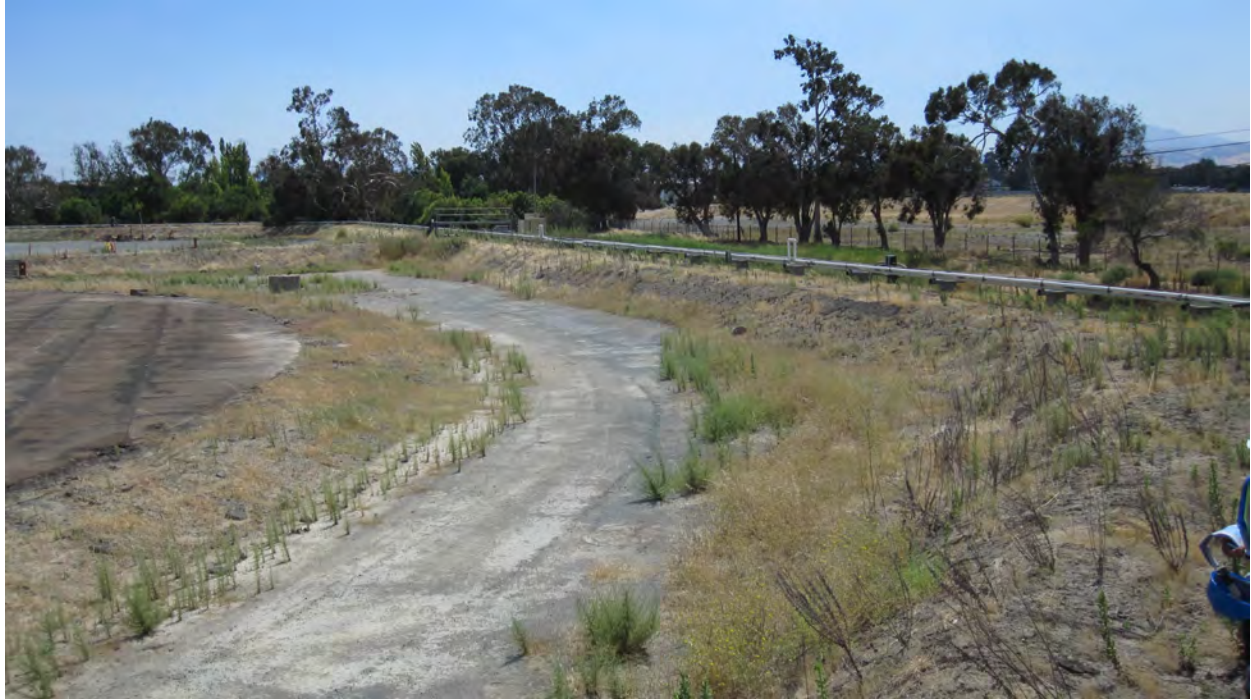
Photo 4C: Looking south-southwest over the west edge of the northermost tank pad. The earthen dike (right and center) provided secondary containment for the former tank farm and will be regraded. Trees in background are inside the Site boundary and will be removed.
