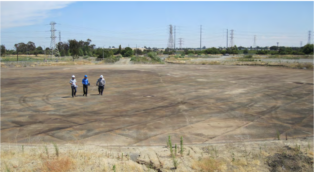
Photo 4B: Looking southeast over the northernmost tank pad. The asphalt surface will be removed by grading. Due to the presence of existing asphalt and concrete surfaces, the proposed project development will reduce the impermeable area onsite compared to existing conditions.
