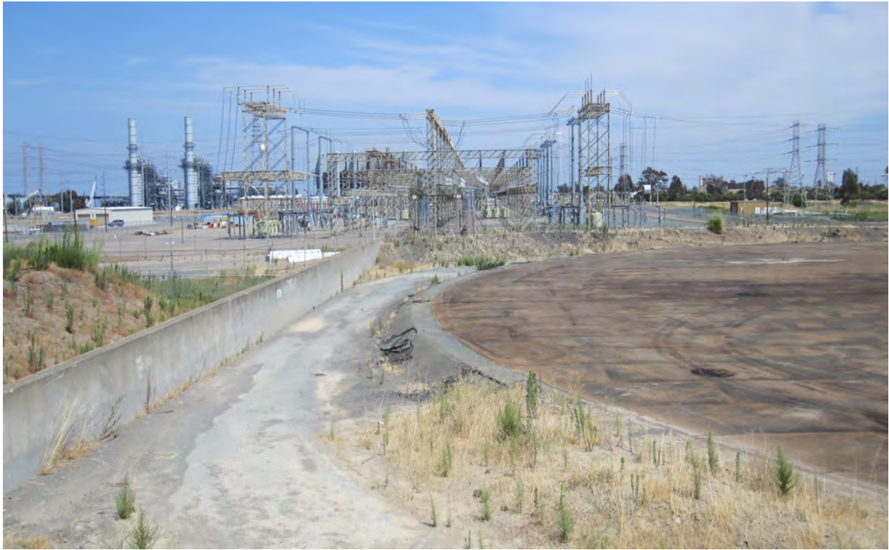
Photo 4A: Looking east along the concrete wall at the north edge of the Site. The asphalt surface of the northernmost tank pad is evident at right. The wall (left and center) provided secondary containment for the former tank farm and will be removed.
