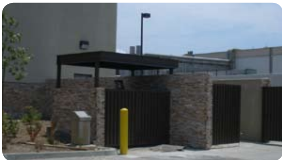
Figure 4.3.6 Refuse areas should be screened and match the overall design of the business park
