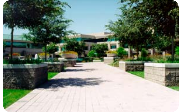
Figure 4.3.4 Well defined pedestrian access connects buildings, parking and transit stops
