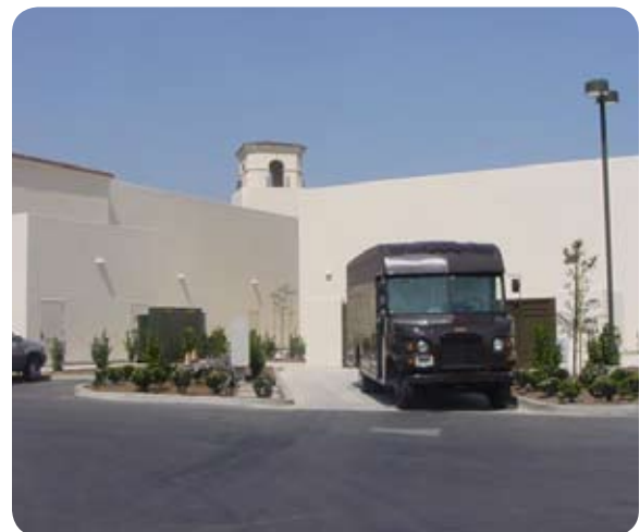
Figure 4.6.1 A loading facility that is screened from public view by placement in the rear of the building
