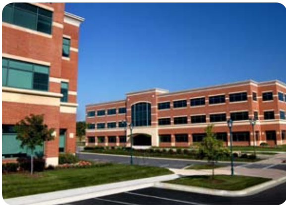
Figure 4.4.1 A business park with a unifying architectural theme
