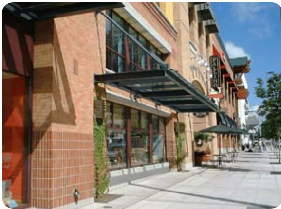
Figure 5.4.9 This building has a well-defined building base with durable materials
