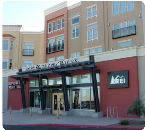
Figure 5.4.4 Upper floors of this building are distinct from the ground floor
