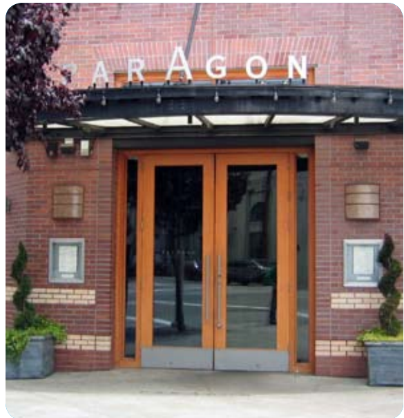
Figure 7.4.8 A projecting sign shall be placed at least 8 feet high and below the first floor ceiling line
