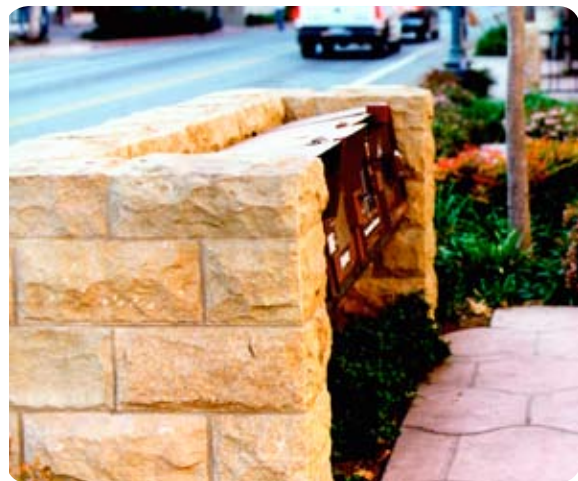
Figure 8.3.9 A screened newspaper rack enclosure limits the number of racks and opens to the sidewalk
