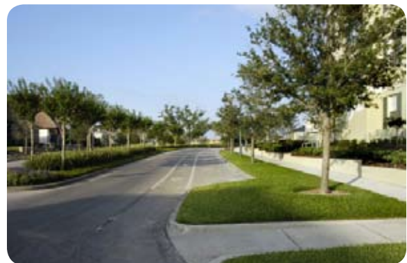
Figure 8.4.4 An example of how a narrow travel lane can slow traffic
