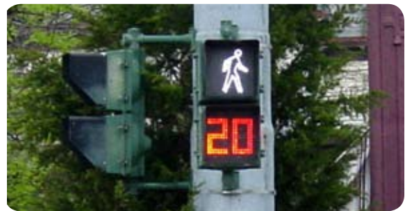
Figure 8.3.5 Crosswalks utilizing countdown signal
