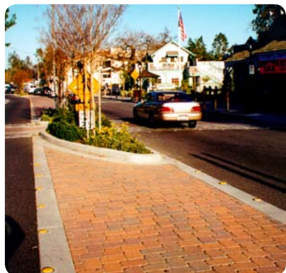
Figure 8.3.18 The pavers in this median contrast with the asphalt in the driving lanes
