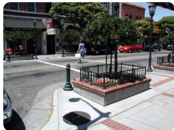
Figure 8.3.4 Types of bulb-outs
