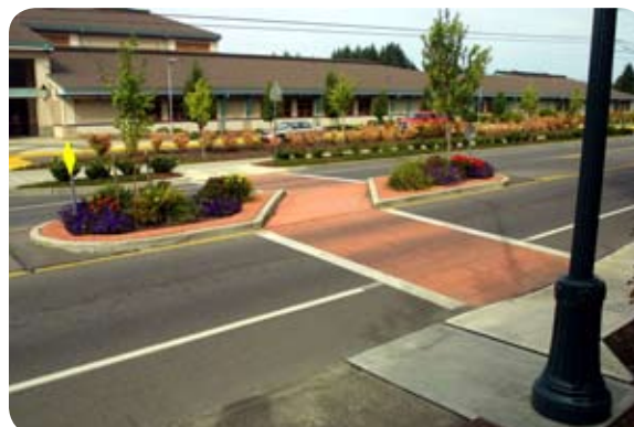
Figure 8.4.2 The color of the crosswalk and refuge island allow the pedestrian areas to stand out
