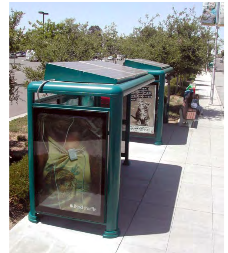
Solar arrays fitted on the roof of the bus stop can power the information displays and the nearby light fixtures.
