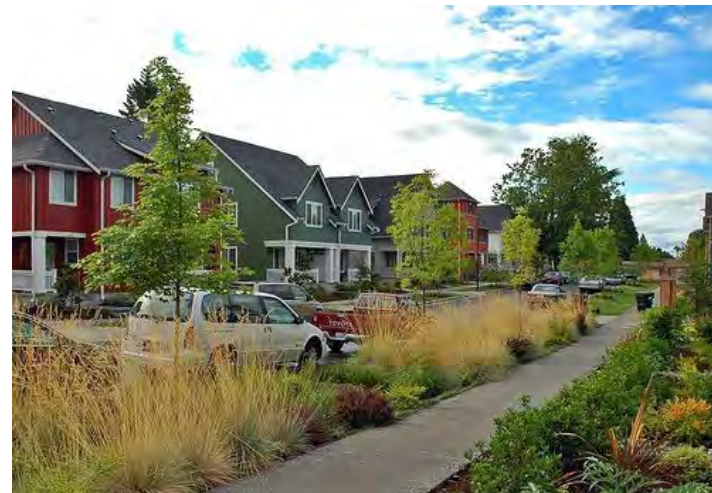
Low impact development (LID) stormwater features such as bioswales, should be maximized to the extent possible.
