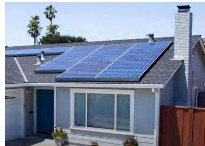
All buildings should be prewired for future solar PV system installation.
