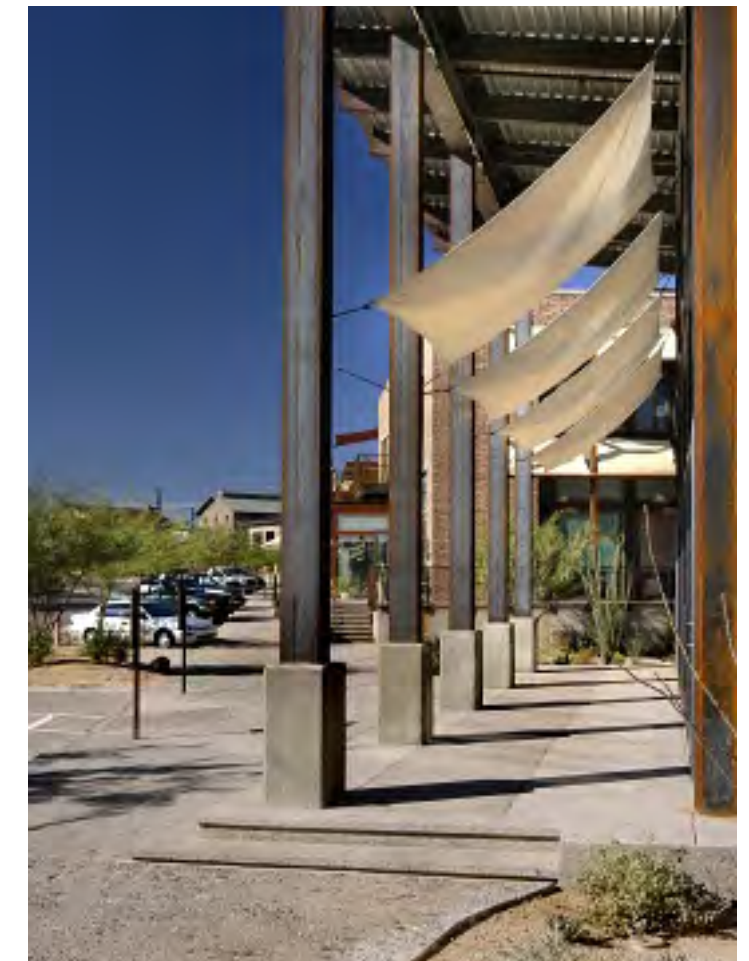
Passive cooling elements can be incorporated into the building design at the Village Center to reduce heat gain.
