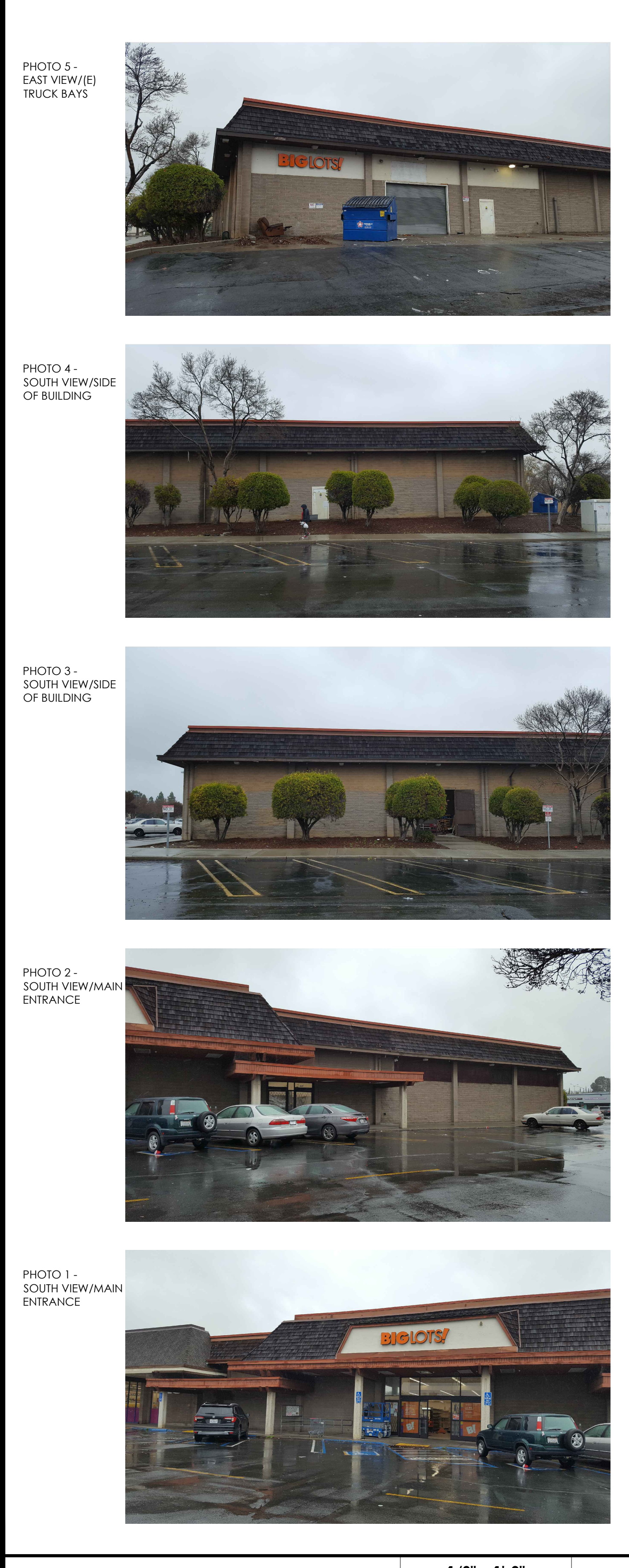
PHOTOS - EXISTING EXTERIOR 1/8" = 1'-0" 01
