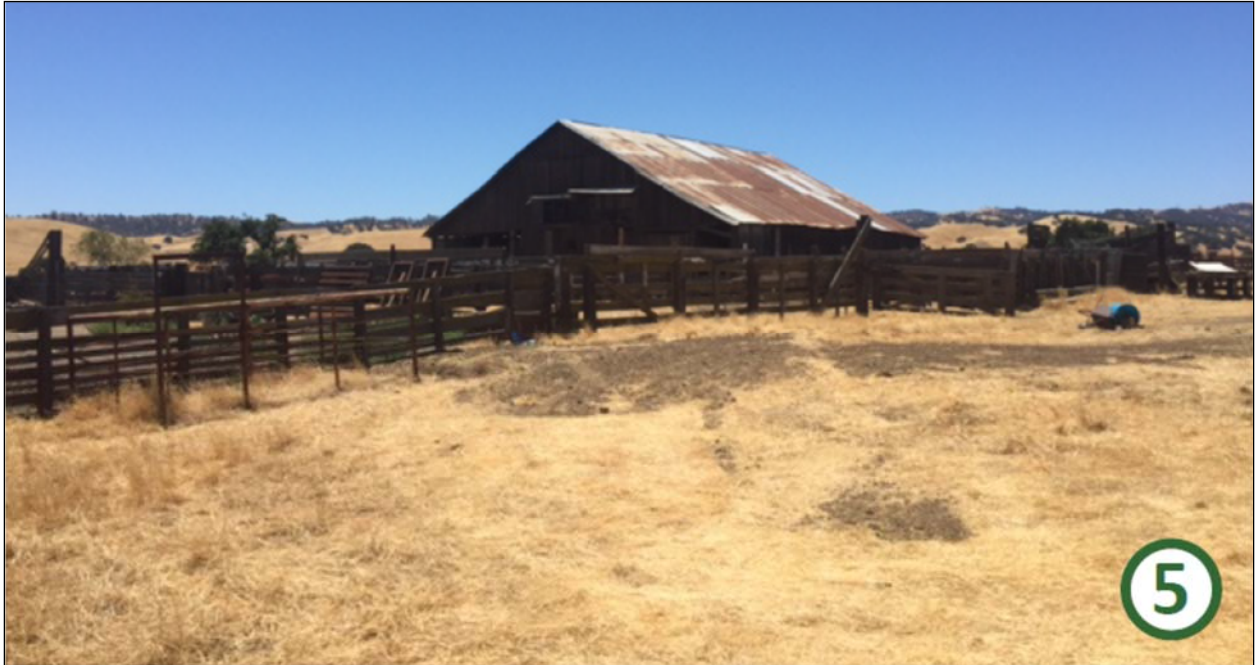
Figure 4.1-6 Existing View from Location 5 – Looking Southwest at the Existing On-Site Barn Structure
