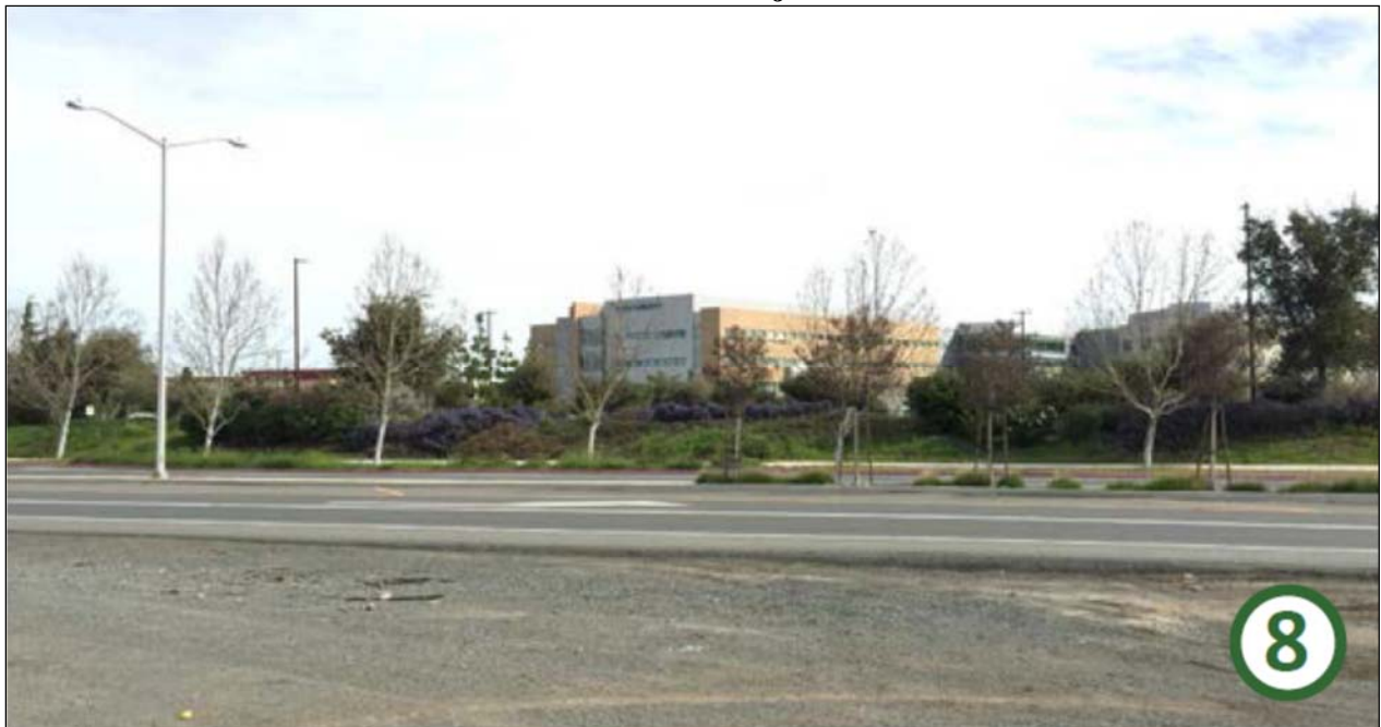
Figure 4.1-9 Existing View from Location 8 – Looking East at Kaiser Permanente Antioch Medical Center from the Project Site
