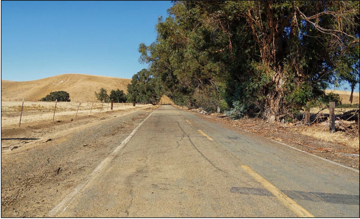
Figure 4.1-13 Existing View Looking North Along Empire Mine Road (View 3)
