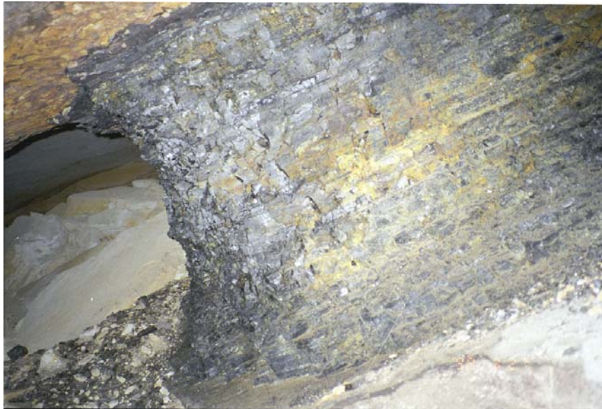
Photo 4: This is the edge of a pillar within a room. This pillar was retreat mined. It is now 6 to 8 feet in diameter. It originally would have been 10 to 15 feet in diameter.
