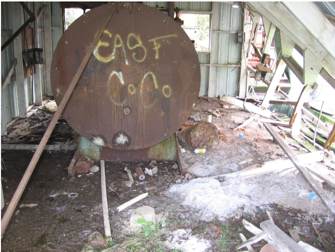
BOILER ROOM IN FEED LOT BUILDINGS
