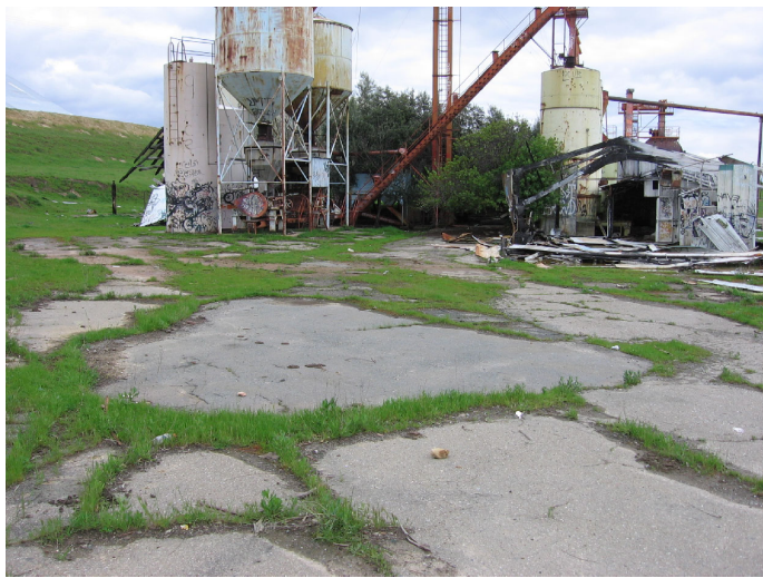
FEED LOT BUILDINGS ON APN 057-060-006
