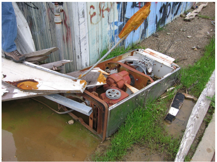
FUEL PUMP AT THE WEST END OF FEED LOT BUILDINGS
