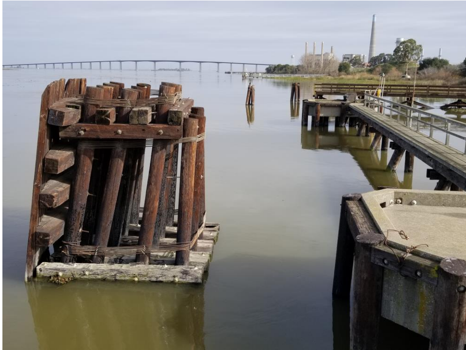
Figure 9. 16-pile Pivot dolphin off east end of wharf and eastern mooring docks.
