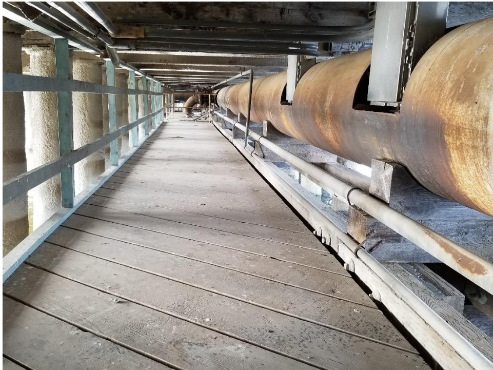
Figure 10. Walkway and pipeline below concrete deck.
