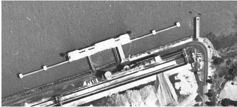
Figure 5. Aerial photographs of the wharf in 1965. Also shown is the onshore pulp receiving facility (courtesy of the Special Research Collections, UCSB Library, University of California Santa Barbara)
