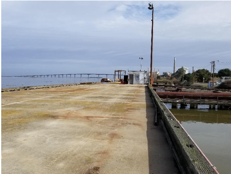
Figure 3. View of main wharf deck, facing east-northeast.
