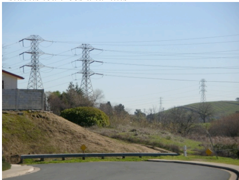
Transmission towers and power lines
