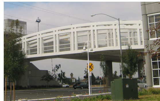
VTA Bridge to Light Rail; Milpitas, CA
