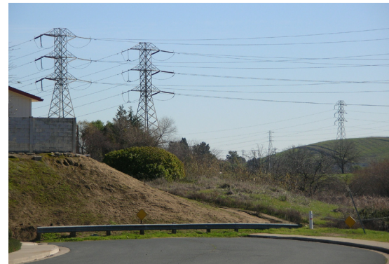
Transmission towers and powerlines.
