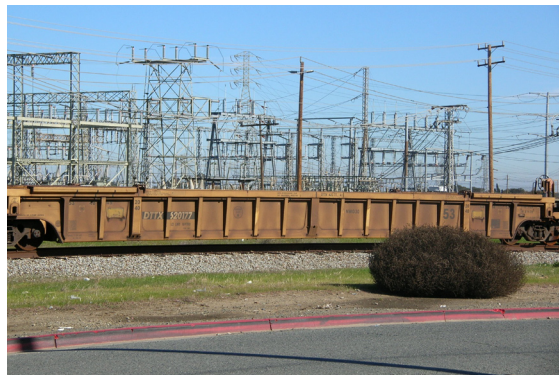
Hillcrest Avenue Substation and rail line.
