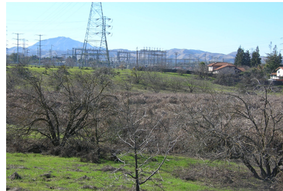
PG&E Substation and an adjacent residential neighborhood.
