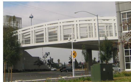
VTA Bridge to Light Rail; Milpitas, CA
