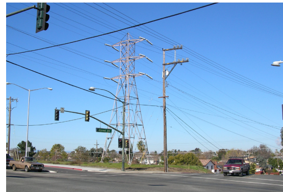
PG&E Overhead Lines: Provide landscape buffers adjacent to the overhead PG&E lines.
