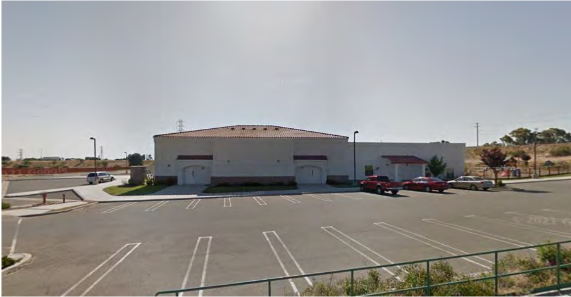
Site 164 | 3415 Oakley Road
