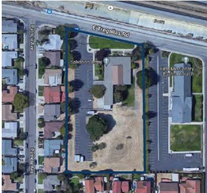
Site 155 | 620 E Tregallas Road
