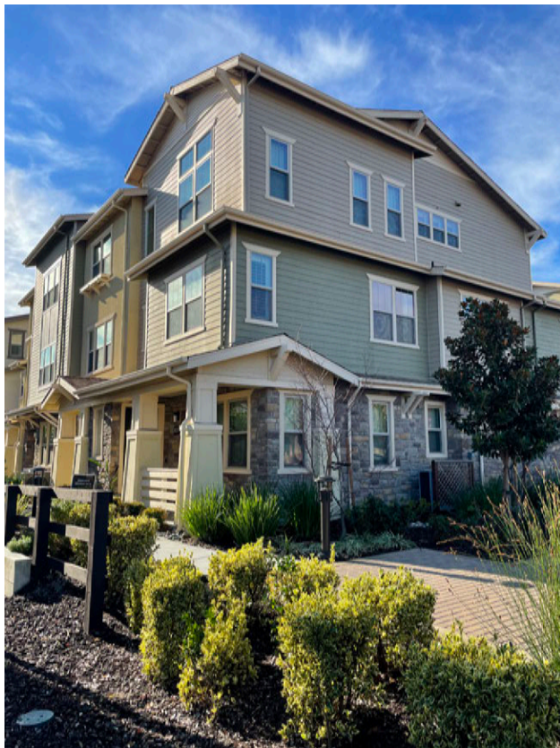
Vertically oriented and proportioned facade openings/windows with divisions.
