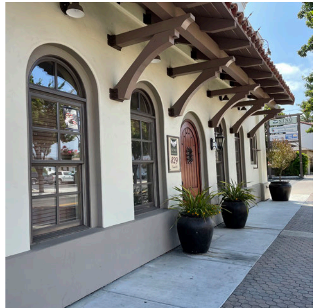
Recessed, vertically oriented and proportioned windows with true divided lite divisions on a street-facing facade.
