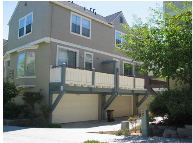
Townhouse balconies projected over garage doors.
