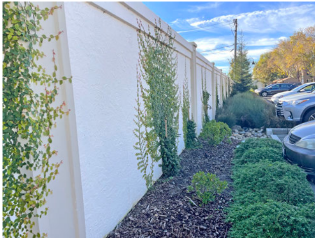
Perimeter wall with decorative columns and landscaping to break up and soften its appearance.
