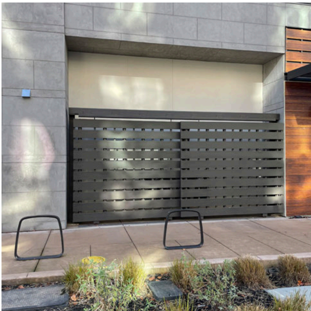
Trash area screened from public view with fencing and gate of matching material and color.
