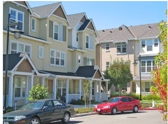
Articulated roof line of a townhouse development.
