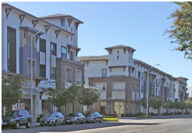
Mixed-use development with bracket details at the cornice and roof eaves; ground floor height of at least 15 feet high; and distinct top, middle, and base.
