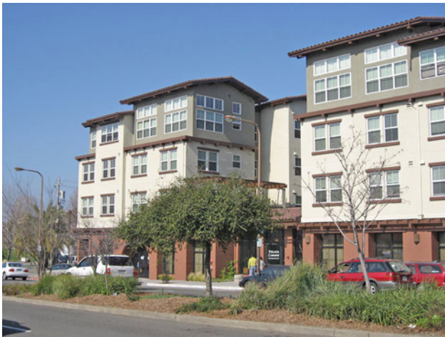
Mixed-use building with varied rooflines to create separate building forms.
