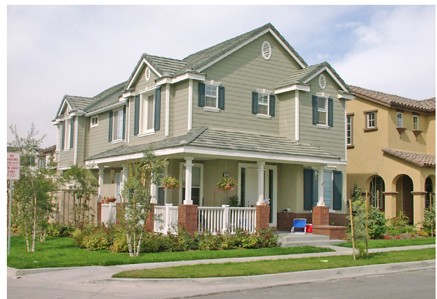
Corner unit with roof gables and wrap-around cladding.
