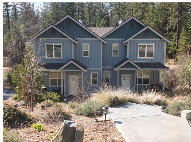
Duplex that highlights the different units through separate roof forms, vertical definition and offset units.
