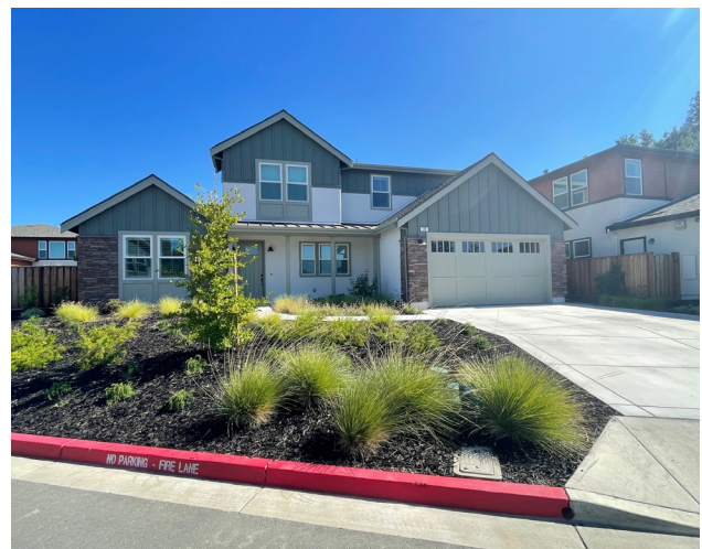
A wide, street-facing roofline with vertical articulation, changes in height and orientation and projecting forms.
