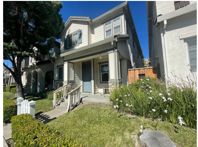
Main entryway porch showing appropriate width, height and compatible materials and colors.
