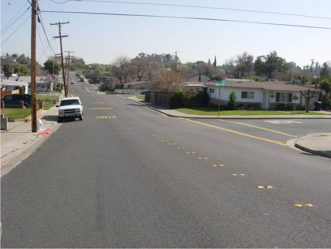
Photo 5: Putnam Street near D Street intersection (looking east).
