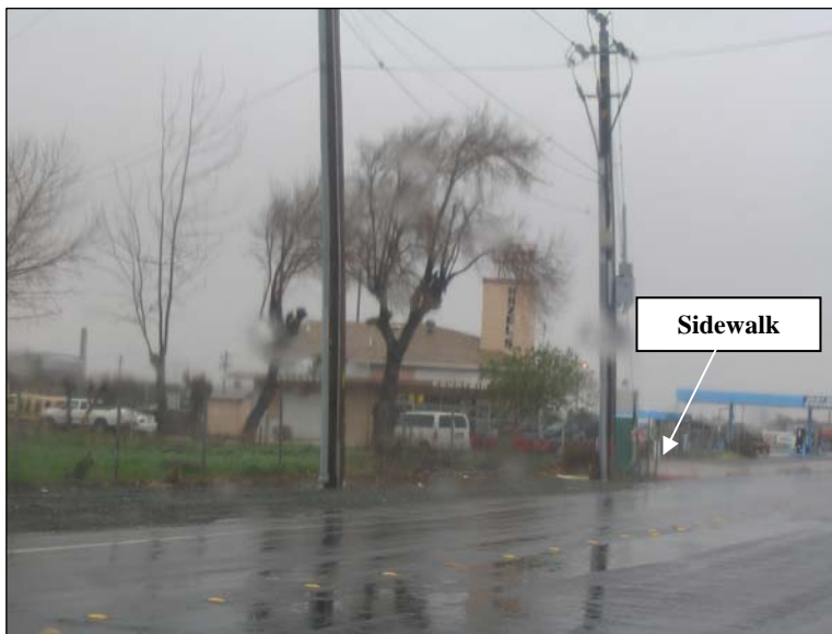
Photo 2: View northeast along Pittsburg-Antioch Hwy. headed towards Auto Center Dr./Somerville Rd.
