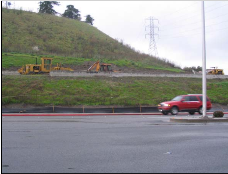
Photo 17: View east at Terranova Dr. and Lone Tree Way intersection showing backhoes on hill and recent foundation.
