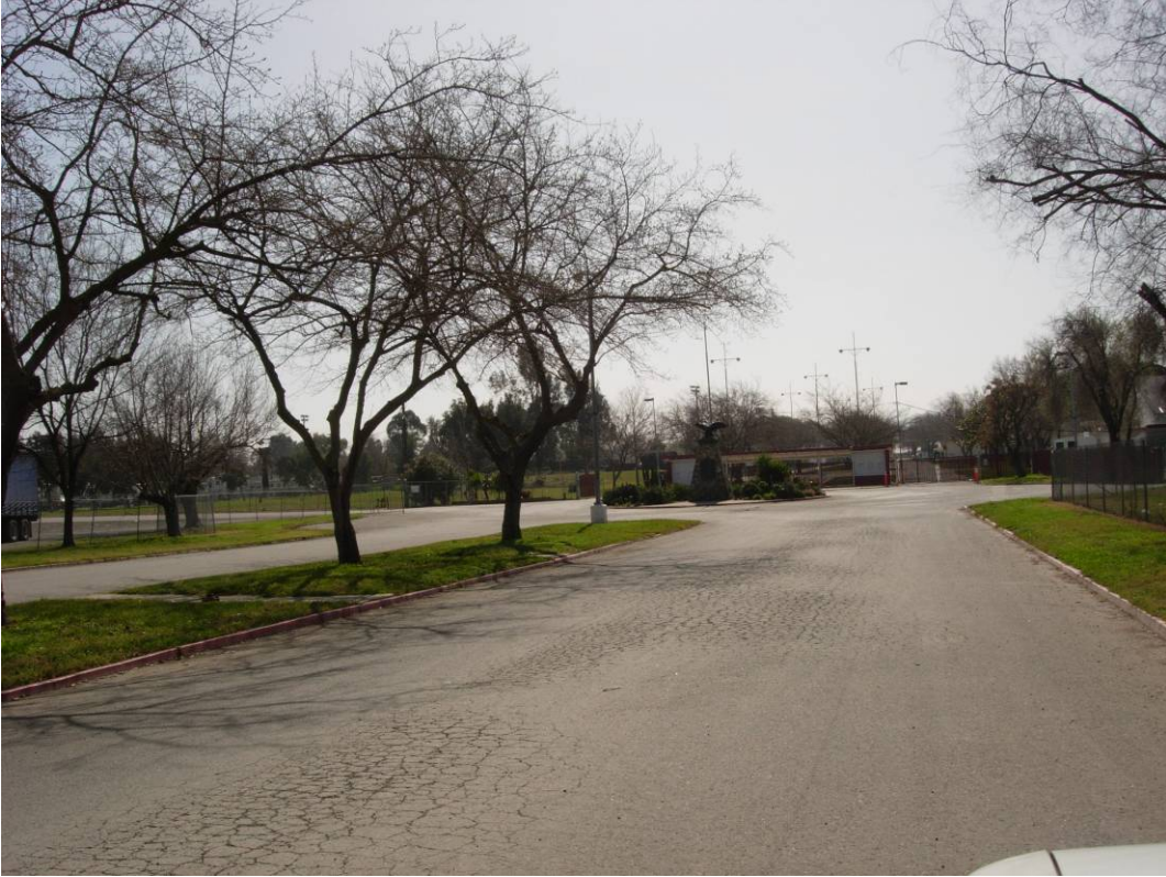
Photo 11: Roadway entrance to Fairgrounds Park
