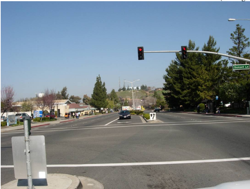
Photo 2: Lone Tree Way at Sunset Lane (looking north).
