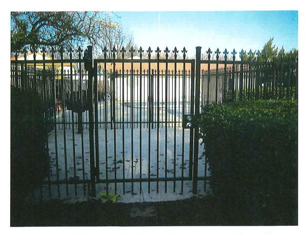
Figure 4: Typical keyed pedestrian access control gate. Gate located at the easterly entrance from Peppertree Way.
