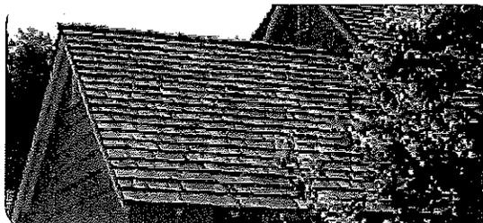
*Figure 6.3.13 Acceptable roofing types include (from top) Asphalt Composition Shingle, Clay Tile and treated Wood Shingle*
