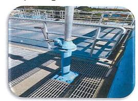
**Project Description:** This project will repair or replace sluice gates, flight drive shafts, housing, and bearings within the basin of Plant "B" at the Water Treatment Plant.
