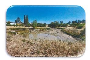
**Project Description:** This project will re-evaluate the existing sludge lagoon. Work included in this project may include removal of accumulated solids, stabilization of banks and installation of decant/disposal system or constructing a new City owned facility.
