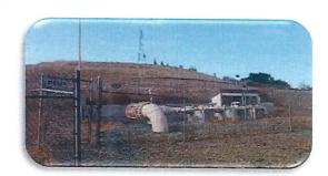
**Project Description:** This project will replace outdated electrical panels, pumps, motors, control valves and install a new flow meter at the Lone Tree Way Booster Pump Station.
