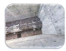
Project Description: This project will replace a deteriorating valve on the raw water line into Plant "A".
