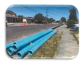
**Project Description:** This project will construct a second pipeline for conveying raw water from the Municipal Reservoir to the Water Treatment Plant.
