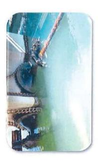
Project Description: This project will replace the existing chains and flights of the sludge collection and removal system for sedimentation basins at Plant "B". Justification: The chain and flight system is a critical system component and prone to significant wear over its constant use and needs to be replaced on a routine basis.
