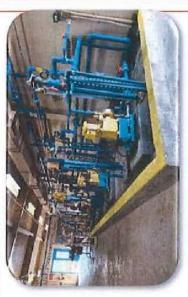
Project Description: This project will install flow paced pump meters and motors for chemical introduction at the Water Treatment
