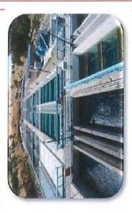
Project Description: This project will replace the granular activated carbon filters of both Plant "A" and "B".
