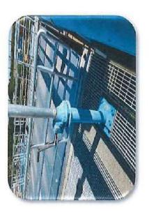
Project Description: This project will repair or replace sluice gates, flight drive shafts, housing, and bearings within the basin of Plant "B" at the Water Treatment Plant.
