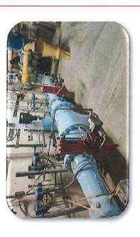
Project Description: This project will replace four aging filter valves in Plant 'A' at the Water Treatment Plant.
