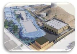
Project Description: This project will construct a 6 MGD brackish water desalination plant that would treat water from the San Joaquin River during times of high chloride content. The work will include the replacement of the City's river intake facility and install a new fish screen. Approximately 4 miles of pipeline will be constructed to convey brine concentrate from the water treatment plant to Delta Diablo.
