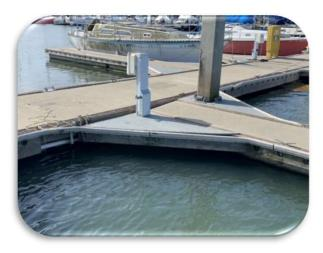
Project Description: This project will replace the docks, floats, and slips at the Marina. Assessments of dock conditions and dive survey to assess the floats will need to be conducted and corner board of slips should be replaced with newer Ultra High Molecular Weight Polyethylene plastic boards.
