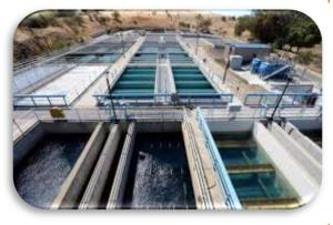
Project Description: This project will replace the granular activated carbon filters of both Plant "A" and "B".
