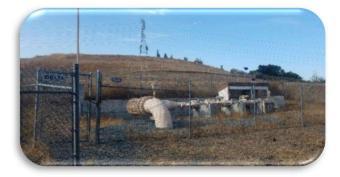
Project Description: This project will replace outdated generator, electrical panels, pumps, motors, control valves and install a new flow meter at the Lone Tree Way Booster Pump Station.
