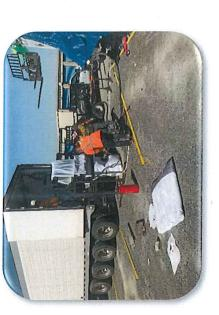
Project Description: The Project will consist of pipe bursting and replacing the old lines through a trenchless sewer replacement method without impacting residents' yards and landscaping.
