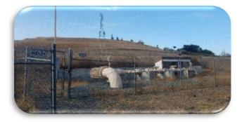
Project Description: This project will replace outdated generator, electrical panels, pumps, motors, control valves and install a new flow meter at the Lone Tree Way Booster Pump Station.
