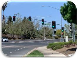
Project Description: This project will improve signal hardware including lenses, backplates with retroflective borders, mounting, size, and number. This will also install pedestrian countdown signal heads and install an advance stop bar before cross walk.
