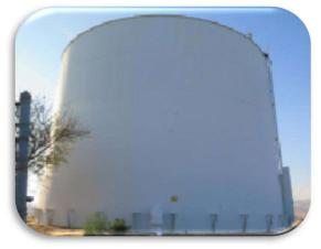
Project Description: This project rehabilitates water storage reservoirs throughout the City. Work to be performed may include recoating, repainting, installation of mixers and sampling stations and seismic upgrades.
