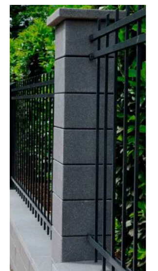
BLOCK PILASTER WITH PRECAST CAP AT MAIN ENTRY.
