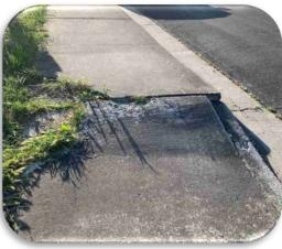
Project Description: This program will replace concrete sidewalks, curb and gutter that have been damaged by tree roots or broken as part of an underground utility repair. The program also installs new curb ramps to improve pedestrian accessibility.
