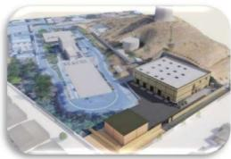
Project Description: This project will construct a 6 MGD brackish water desalination plant that would treat water from the San Joaquin River during times of high chloride content. The work will include the replacement of the City's river intake facility and install a new fish screen. Approximately 4 miles of pipeline will be constructed to convey brine concentrate from the water treatment plant to Delta Diablo.
