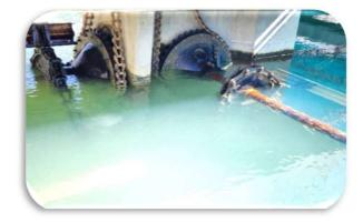
Project Description: This project will replace the existing chains and flights of the sludge collection and removal system for sedimentation basins at Plant "B".
