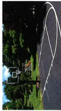
Basketball Court w/ Asphalt Paving (BAYSO NCAA)
