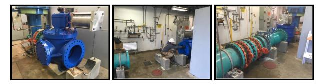
**The Water Treatment Plant** replaced a 20-inch rotary ball valve at the river pump station. The river pump is an essential asset to the City's water resources. When river water meets quality standards, we are able to draw from it as a source of raw water.
