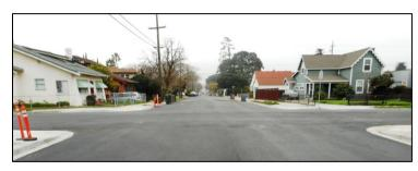
completely rebuilt to improve storm water drainage and pedestrian access. Twenty-four curb ramps were constructed and numerous improvements were made to deteriorating, damaged and uneven concrete flatwork within the project area.
