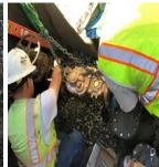
The Water Distribution Division of Public Works is responsible for maintaining the City's treated and raw water distribution systems in safe and serviceable condition. The system delivers treated water to residential, commercial and irrigation customers. In this Weekly Update edition, eight (8) Water Distribution Operators from three (3) different crews worked together to replace four-4" meters and two-10"
