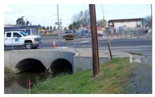
Construction has commenced on the West Antioch Creek Channel Improvements project located near the intersection of West 10th and 'O' Streets. This project will include expanding an under capacity portion of the channel between West 8th and West 10th Streets to reduce the chronic, localized flooding in this area. The existing undersized arch culverts under West 10th Street will be replaced with a larger
