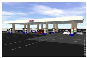
expansion is designed to match the existing structure and will include a tan, metal-wrapped canopy fascia with a cornice and CMU wrapped canopy columns. This expansion will reduce lines and make it more convenient to purchase gas from Costco.
