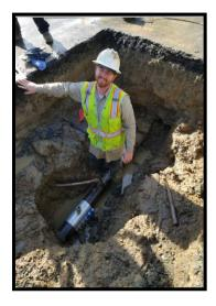
Water Distribution Operators John S. and Simon K. responded to a water break on Belle Drive on Tuesday. The Crew's first priority is to secure the area for public safety. The next priority is to isolate the broken section of the water main to minimize damages and potential of a sink hole from forming as a result of the volume of water. The entire crew worked diligently to restore water service to the affected customers as guickly as possible.
