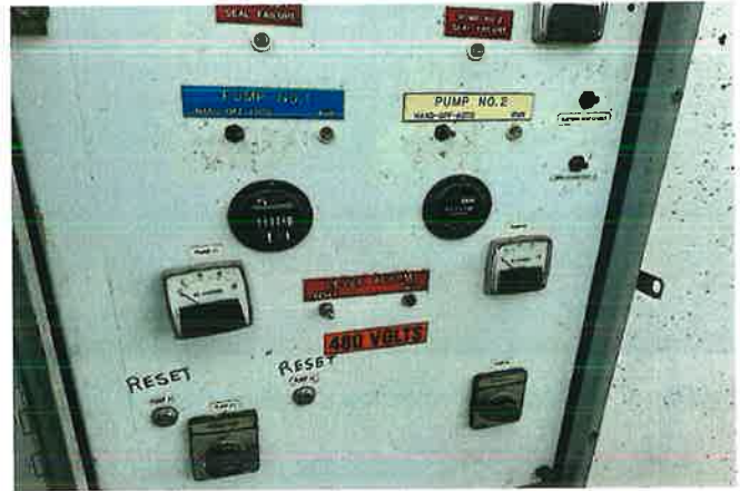
Location D (Photo 2): Pump station motor control panel.
